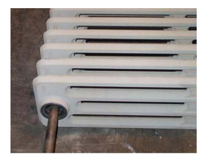
By turning the nipple key, rotate the nipple so that it pulls the 2 radiator assemblies together. At this stage only rotate the nipple by one turn.
