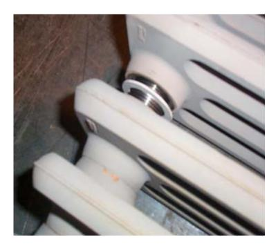
Gently slide the second radiator assembly next to these nipples, ensuring that the thread orientations are correct.
