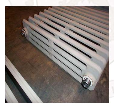
Screw in a pair of nipples to one end of the radiator assemblies.
