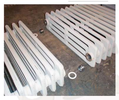
Place the radiator sections to be joined onto a clean, firm and flat surface, ensuring that the machined faces and internal threads are perfectly clean. Each radiator section has right-hand threaded connections at one end and left-hand threaded connections at the other. The nipples have one end left-handed and one end right-handed. For correct assembly you will need to identify the orientation of the connections on the radiator assemblies.
